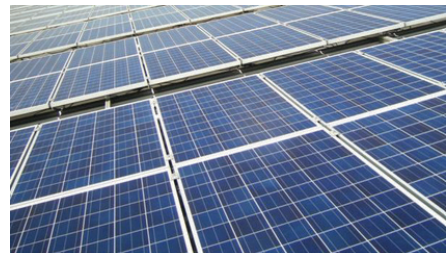
Fitting of Solar Panel Upgrade:
